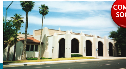
Glendale Civic Auditorium
